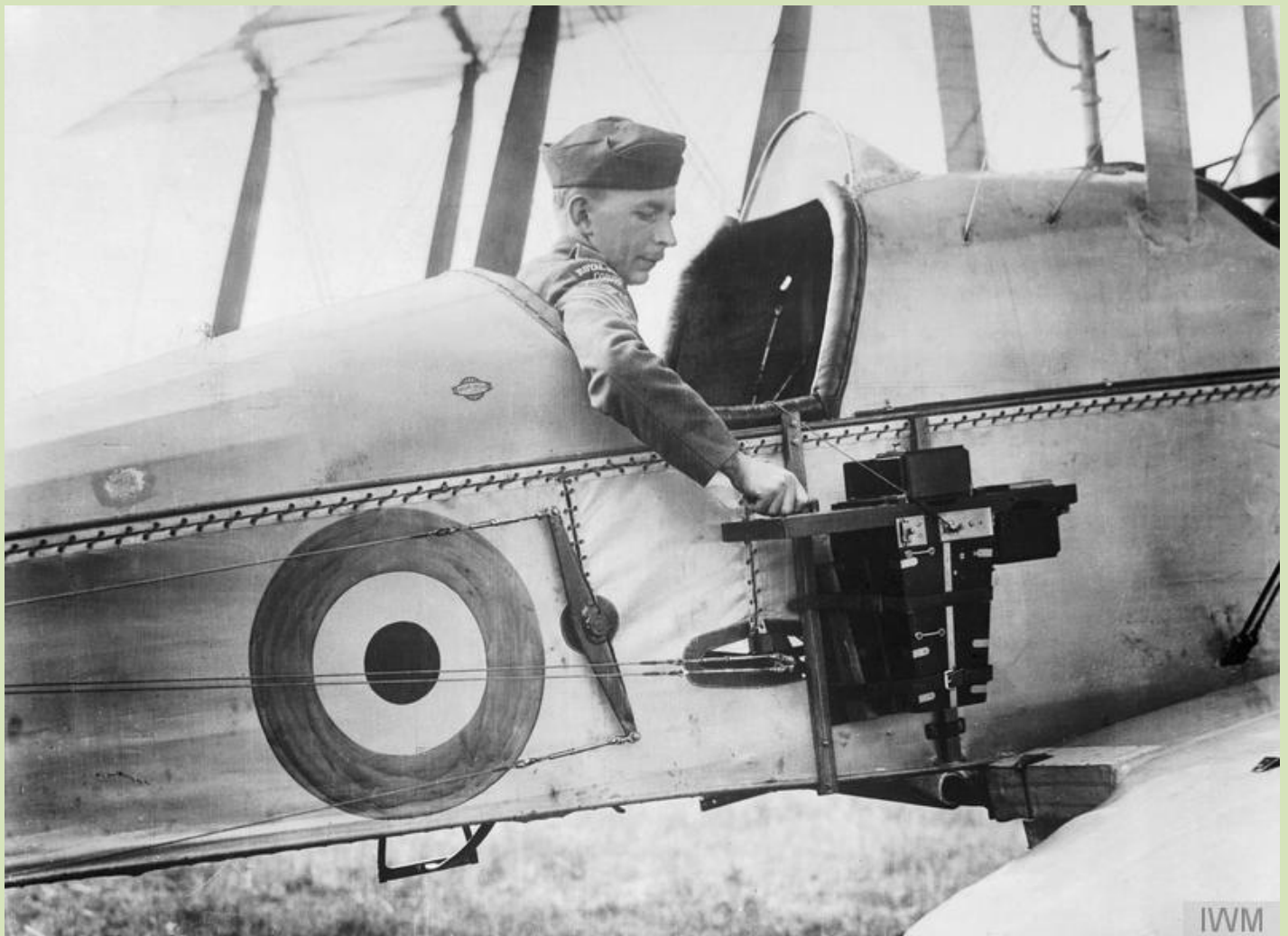
A sergeant of the Royal Flying Corps demonstrates a C type aerial reconnaissance camera fixed to the fuselage of a BE2c aircraft, 1916. Q33850.jpg
